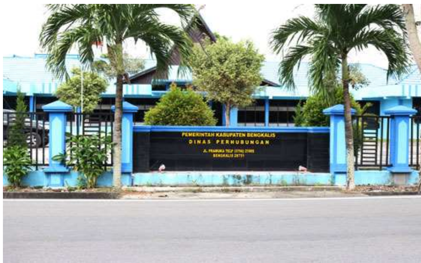
Figure 2. 2 Transportation Department of Bengkulu Regency Office
