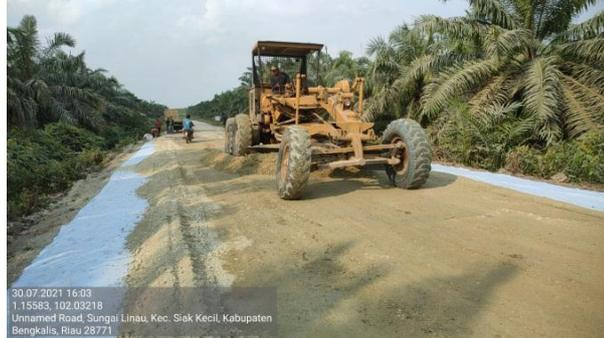
*Gambar 3.8.5 Motor Grader*
