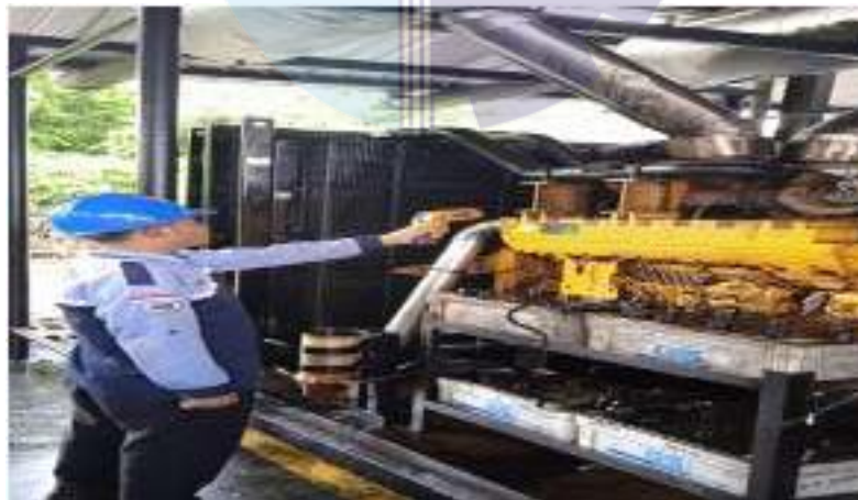
Gambar 2.14 monitoring kwh ( Sumber : PT.MEGAPOWER MAKMUR Tbk.2021)
