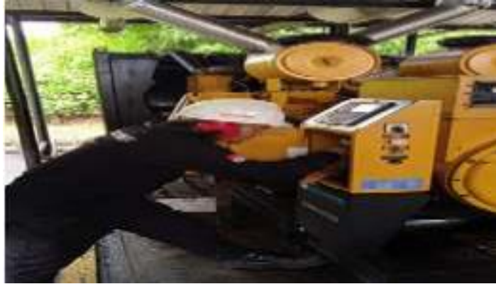
Gambar 2.3 monitoring kwh ( Sumber : PT.MEGAPOWER MAKMUR Tbk.2021)
