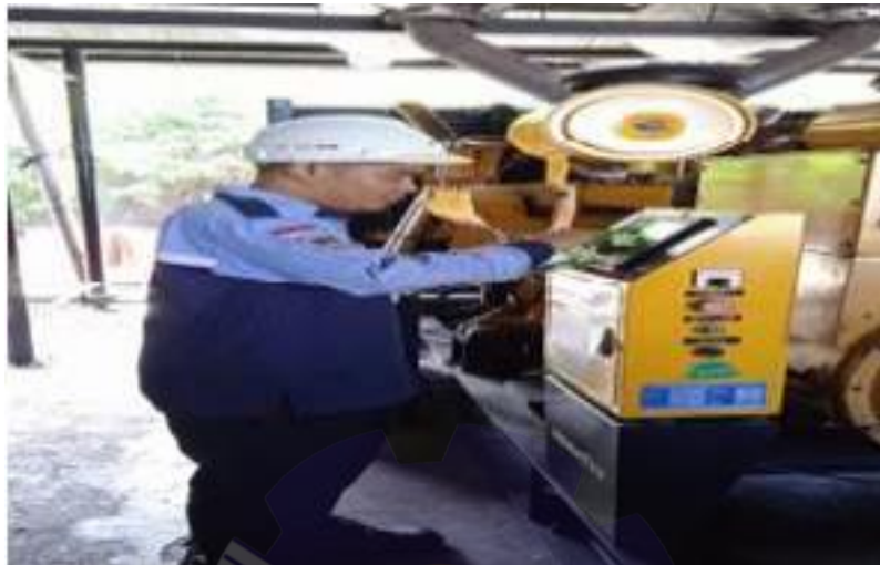
Gambar 2.21 monitoring kwh ( Sumber :PT.MEGAPOWER MAKMUR Tbk.2021)
