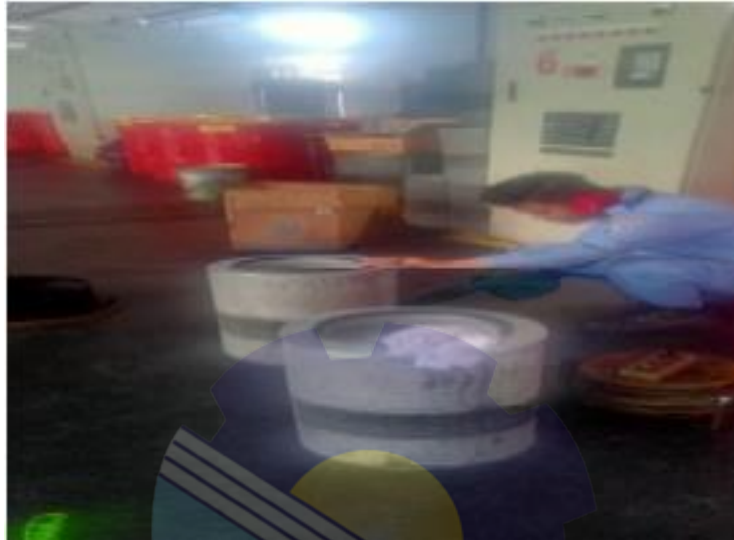
Gambar 2.15 Service filter hawa ( Sumber :PT.MEGAPOWER MAKMUR Tbk.2021)
