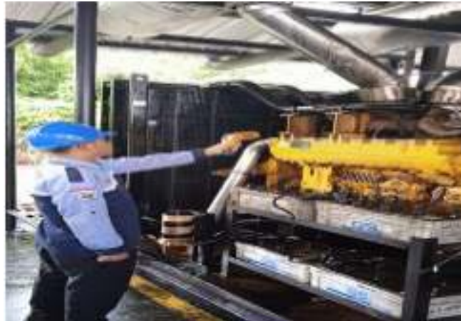
Gambar 2.9 Monitoring Kwh ( Sumber : PT.MEGAPOWER MAKMUR Tbk.2021)
