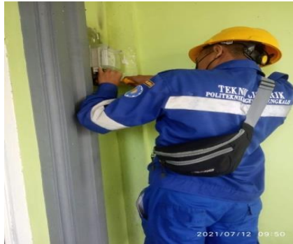
Gambar 2.7 pergantian Kwh meter
