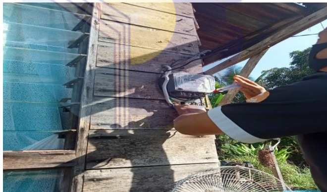
Gambar 2.4 pergantian Kwh meter
