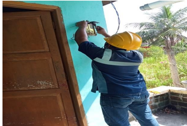
Gambar 2.5 pergantian Kwh meter
