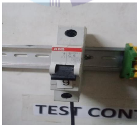
Gambar 3.4 Miniature circuit breaker/MCB
