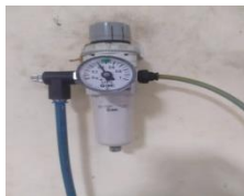
Gambar 2.4 Air regulator, Gambar 2.5 positioner, Gambar 2.6 injector/dcs
