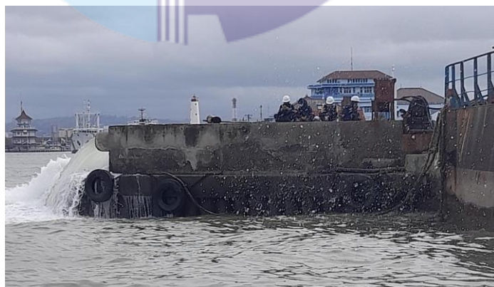
Gambar 2.32 Proses Pengeringan Kolam Graving Dock
