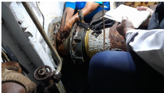
Gambar 2.15 Pengecekan Clearance Intermediate Shaft KMP Kirana III
