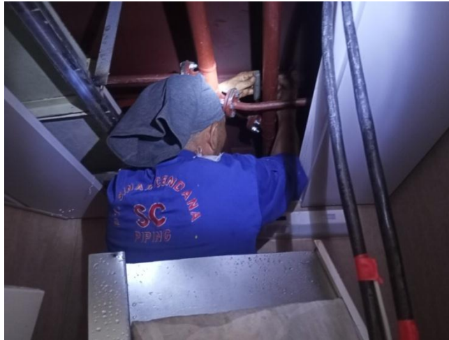
Gambar 2. 69 Repair perpipaan dikamar mandi
