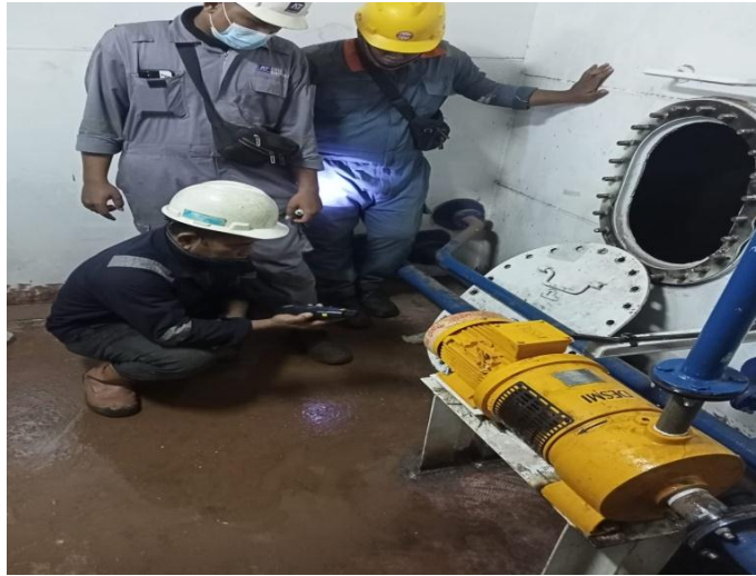
Gambar 2. 16 Commissioning fresh water pump
