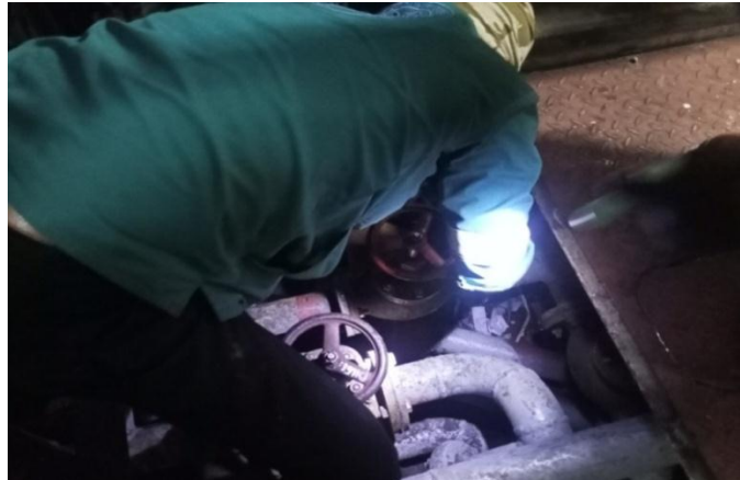
Gambar 2. 67 Repair valve di manifold bilge
