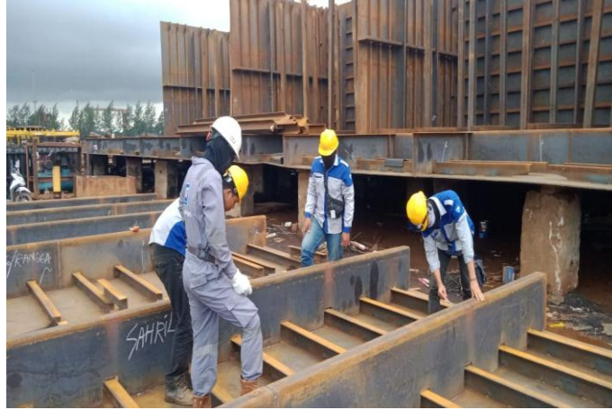
Gambar 2. 7 Inspect welding terhadap longitudinal bulkhead
