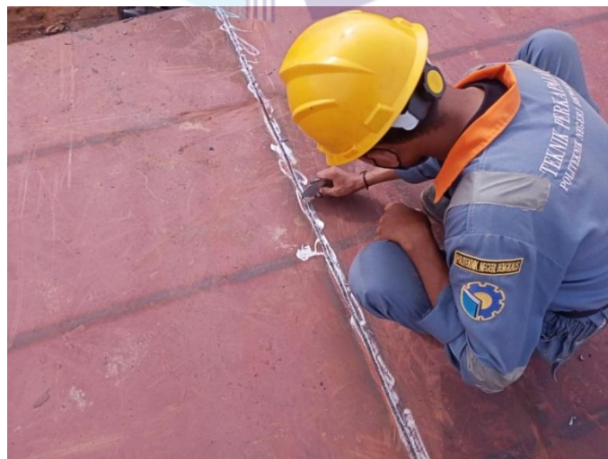
Gambar 2. 58 Pengukuran welding gauge
