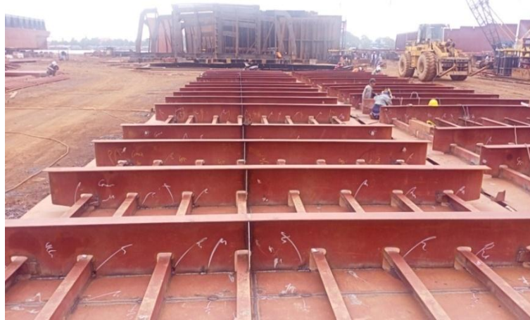
Gambar 2. 40 Inspect welding terhadap long bulkhead
