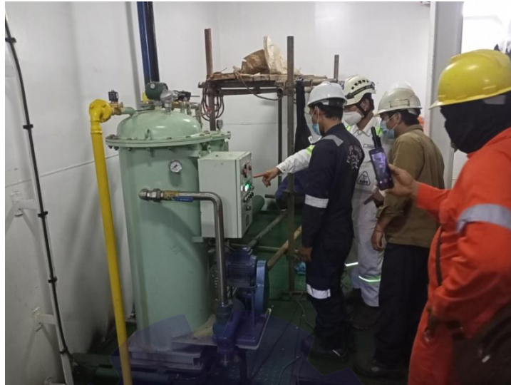
Gambar 2. 60 Commissioning terhadap sistem OWS
