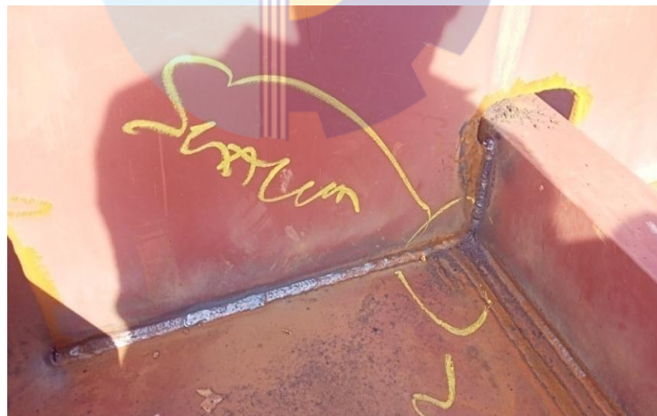
Gambar 2. 41 Inspect welding long bulkhead
