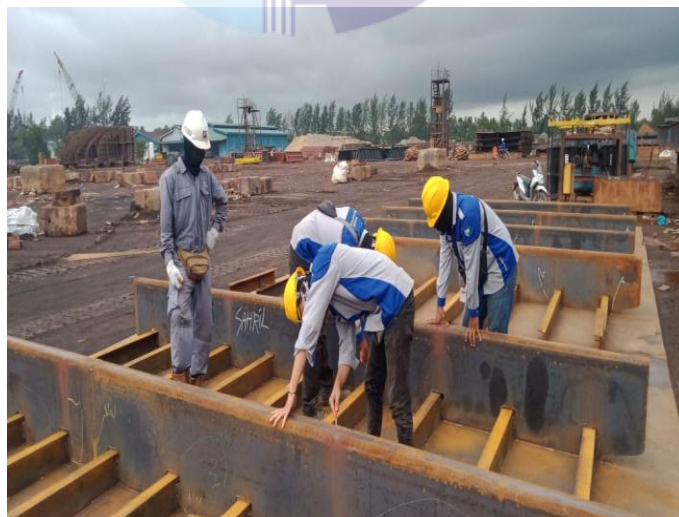
Gambar 2. 9 Inspect welding dibagian bulkhead
