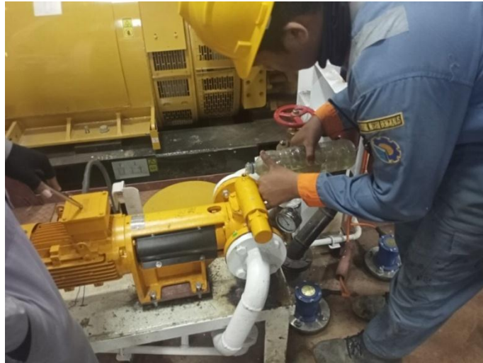
Gambar 2. 26 Commissioning terhadap dirty oil pump
