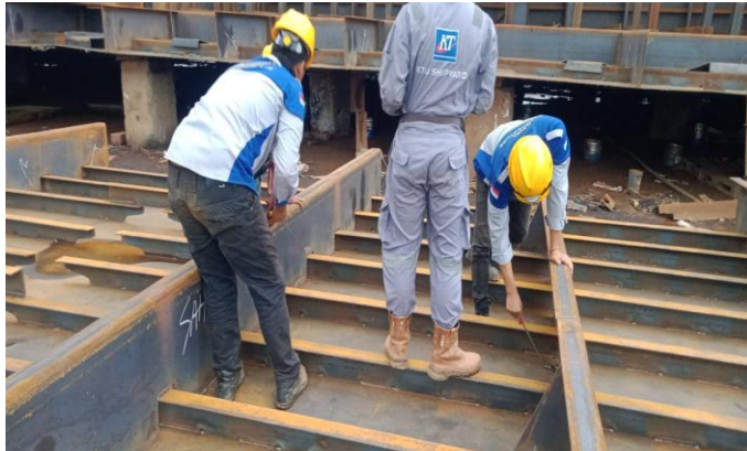
Gambar 2. 10 Inspect welding terhadap bulkhead
