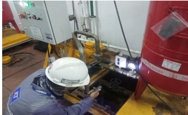
Gambar 2. 25 Pengecekan terhadap tekanan sistem fresh water pump
