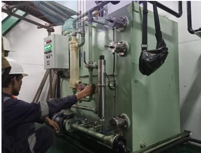
Gambar 2. 62 Commissioning terhadap sistem STP
