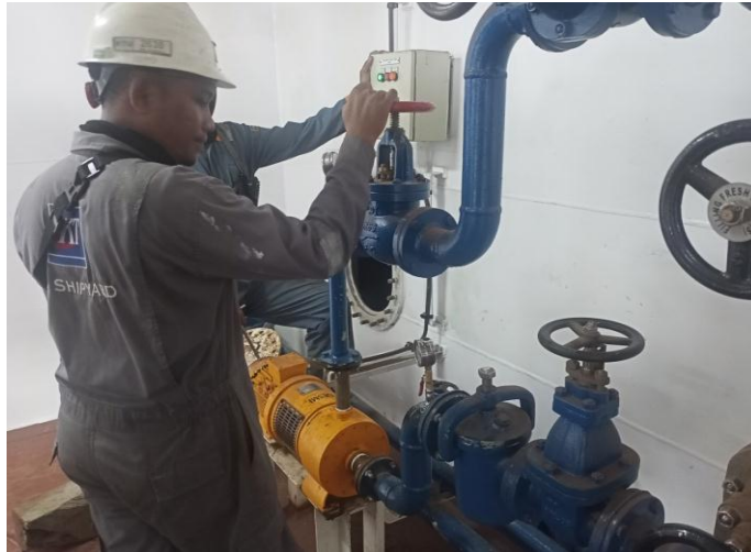
Gambar 2. 23 Pengoperasian mesin fresh water pump
