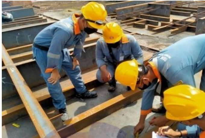
Gambar 2. 3 Proses inspect welding terhadap transverse bulkhead
