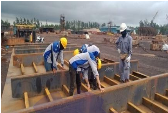
Gambar 2. 5 Inspect welding terhadap longitudinal bulkhead
