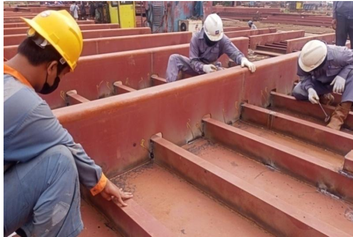
Gambar 2. 38 Inspect welding bottom frame 34-21
