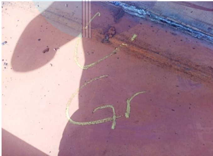
Gambar 2. 36 Hasil inspect welding
