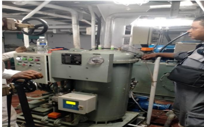
Gambar 2. 74 Commissioning oil water separator
