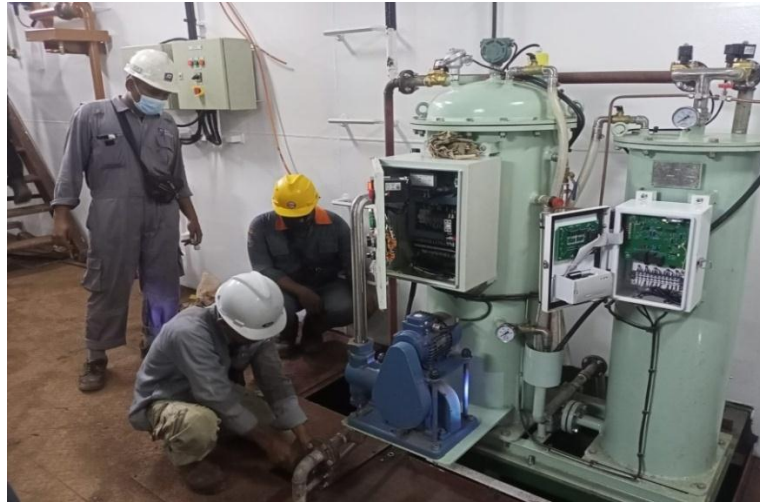
Gambar 2. 19 Commissioning terhadap oil water separator
