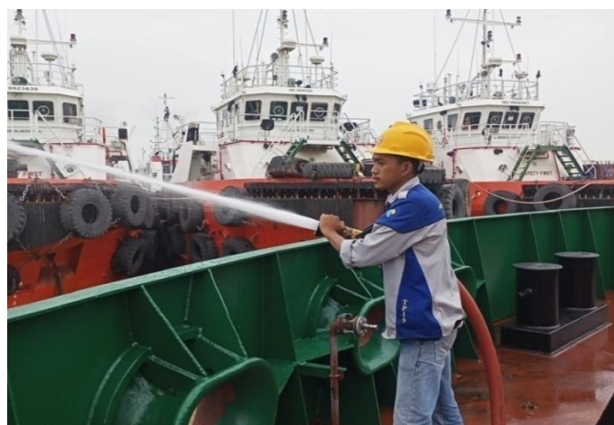
Gambar 2. 49 Commissioning terhadap fire hydrant
