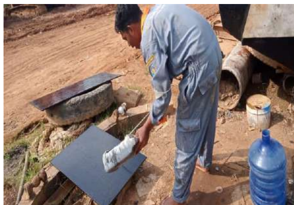
Gambar 2.56 Pengecatan lantai speed boat
