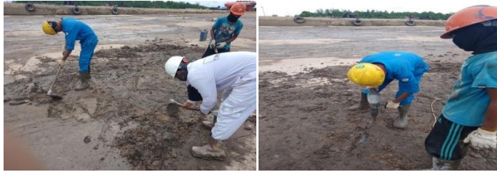
Gambar 2.34 Repair Kolam Slipway 2
