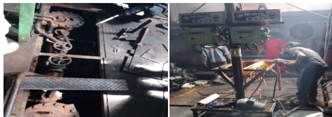
Gambar 2.16 Pengamatan repair ruang mesin tugboat satia samudera 07
