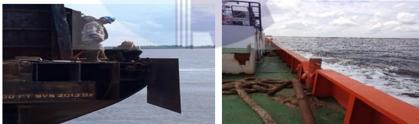
Gambar 2.45 Pengamatan repair tongkang Solid 2 & Sea trial
