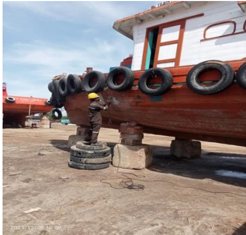
Gambar 2.34 Proses Repair laminasi tugboat Bintang Sejahtera
