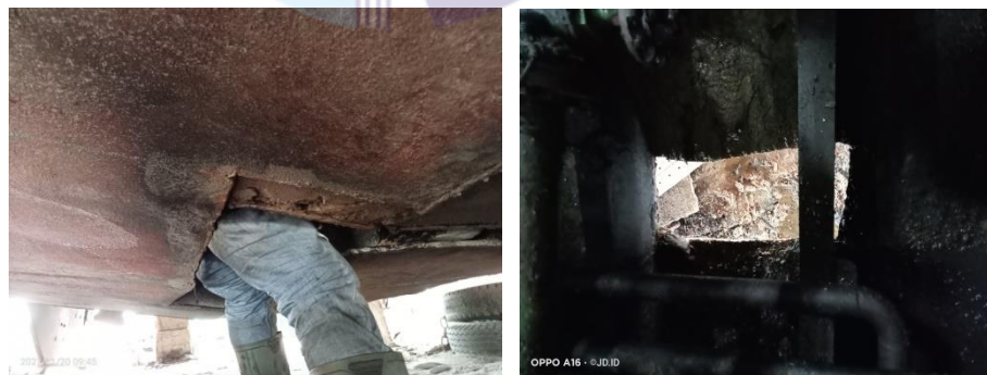
Gambar 2.13 Proses replating bukaan kulit dasar tugboat nelly 19
