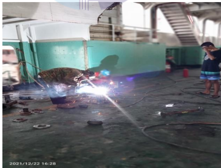
Gambar 2.31 pengelasan pipa Cooler Main Engine
