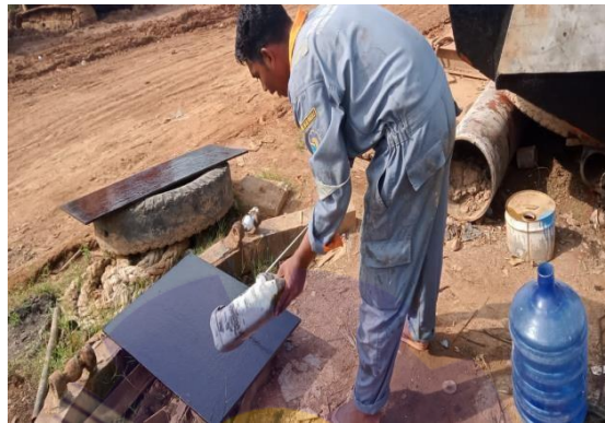
Gambar 2.57 Pengecatan lantai speed boat
