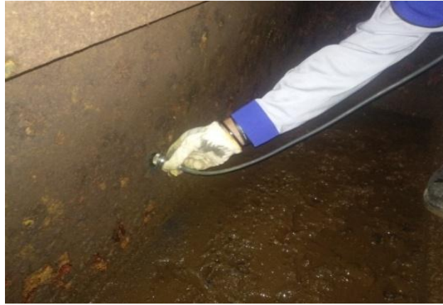
Gambar 2. 12 Ultrasonic Test (UT) Tongkang HAIHANG 1 bagian tank foild Startboard side
