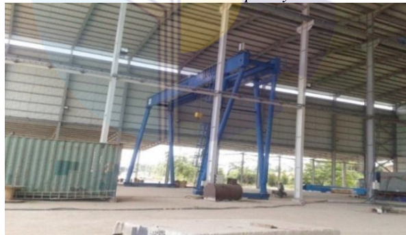
Gambar 1. 2 Main Workshop Fabrication
