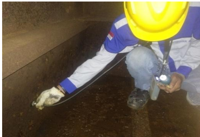
Gambar 2. 11 Ultrasonic Test (UT) Tongkang HAI HANG 1 bagian tank foild Portside
