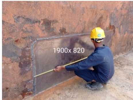
Gambar 2. 60 Insert Plate Sideboard
