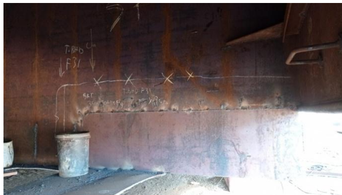
Gambar 2. 50 Insert Plate Trans BHD
