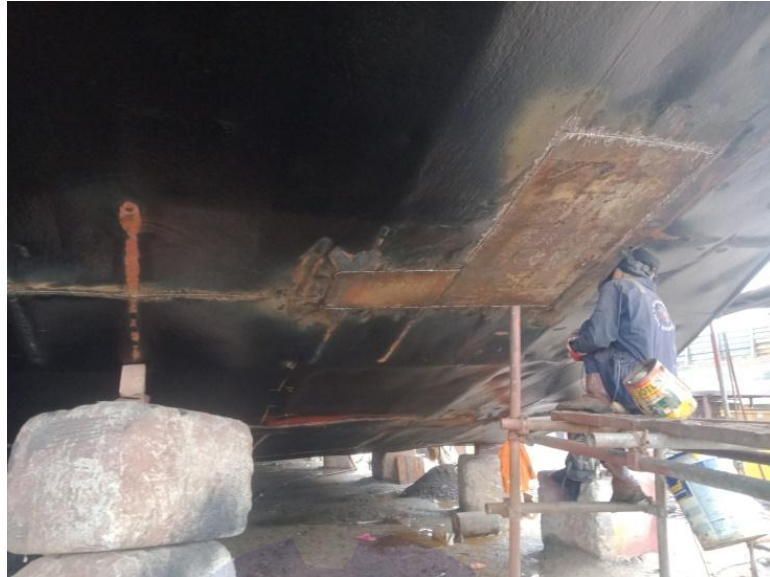
Gambar 2. 39 Replating area Tongkang MONTENGO BAY
