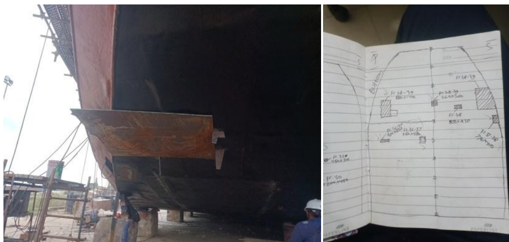
Gambar 2. 38 Replating area Bottom Tongkang MONTENGO BAY
