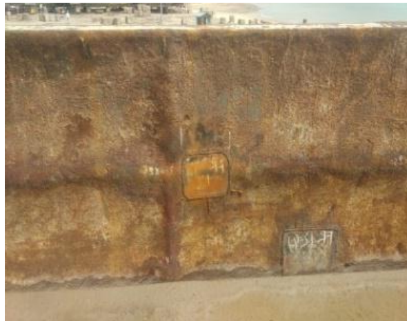
Gambar 2. 14 Replating Area Sideboard
