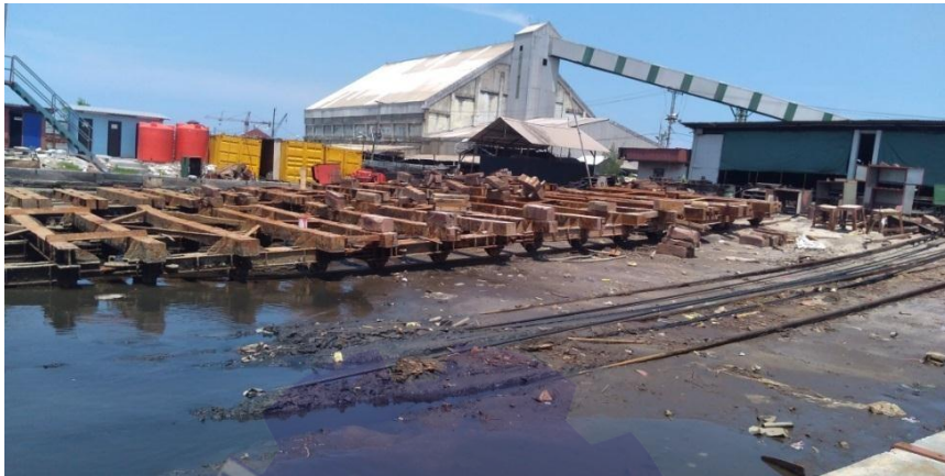
GAMBAR 1.4. Slipway B (Sumber : PT.Yasa Wahana Tirta Samudera)
