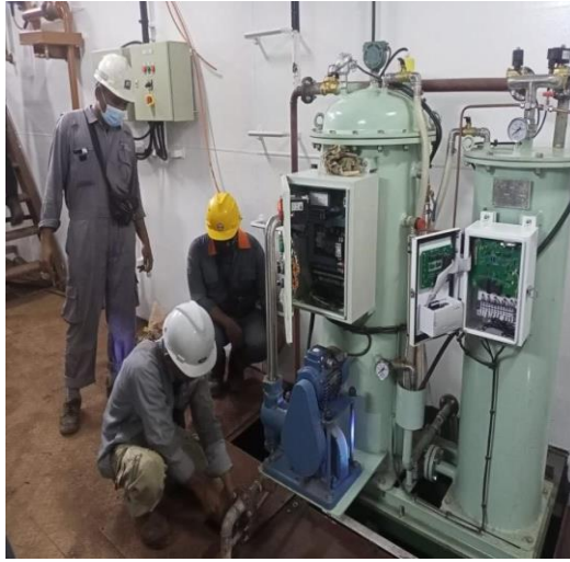
Gambar 2. 20 Pengecekan oil water separator
