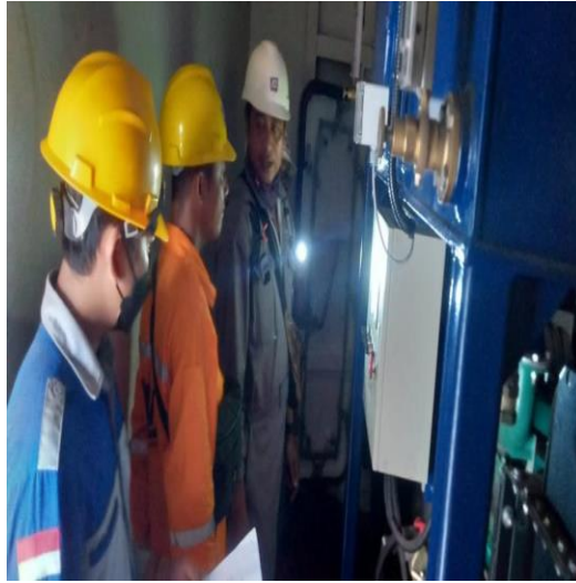
Gambar 2. 29 Commisioning safety device engine windlass
