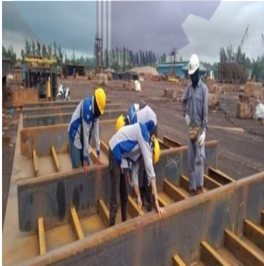
Gambar 2. 5 Inspect wellding longitudinal bulkhead
