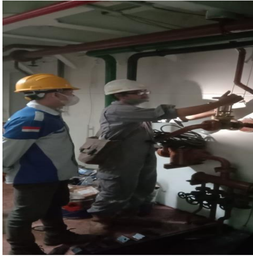
Gambar 2. 32 Membuka quick closing valve
