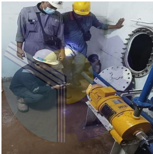
Gambar 2. 17 Commisioning pompa fresh water
