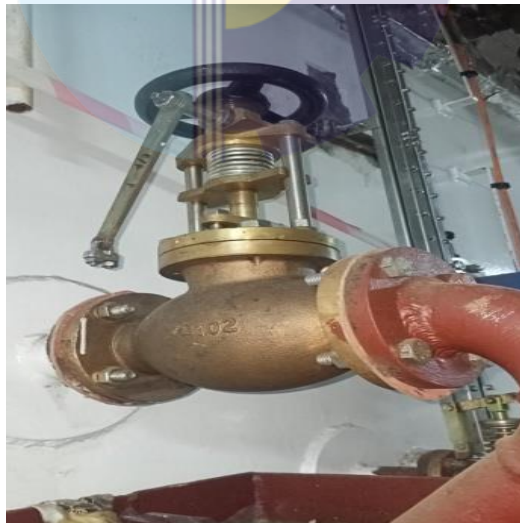
Gambar 2. 8 Contoh gambar quick valve
