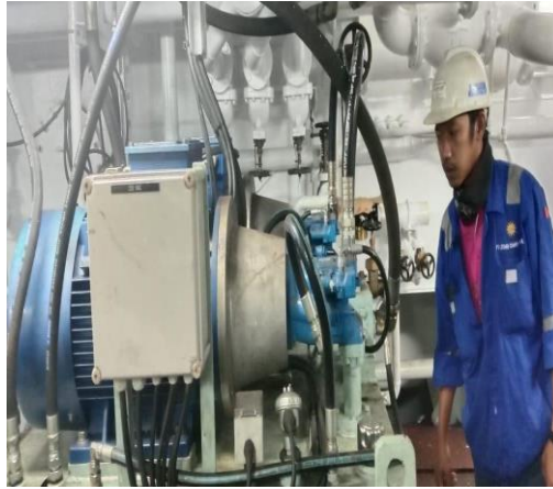
Gambar 2. 38 Commisioning mesin hidrolik towing winch
