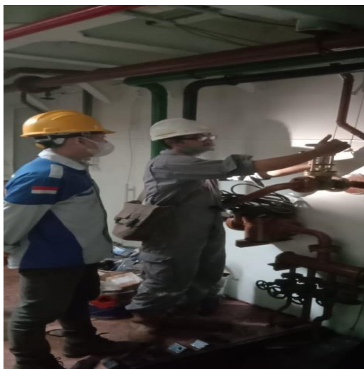
Gambar 2. 32 Membuka quick closing valve
