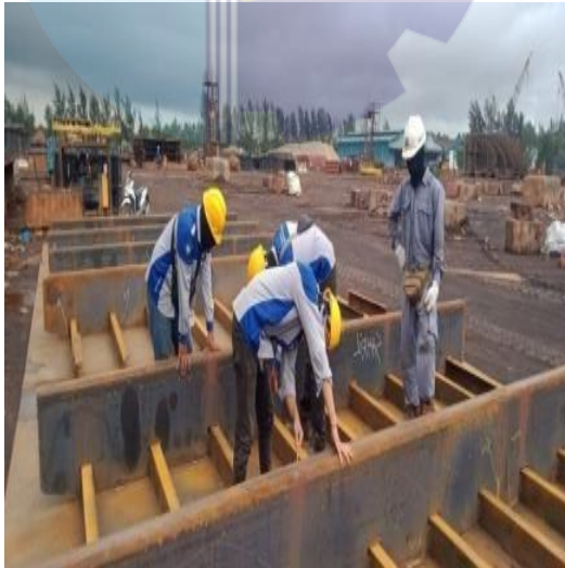
Gambar 2. 5 Inspect wellding longitudinal bulkhead
