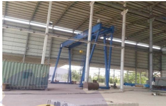
Gambar 1.3 Main Workshop Fabrication
