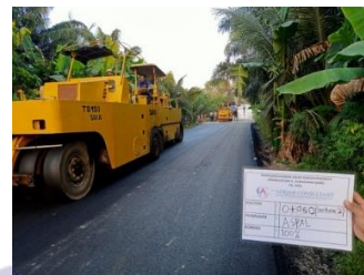
Gambar 2.4 Pneumatic tyred roller
