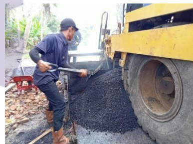
Gambar 2.2 Proses penghamparan Aspal
