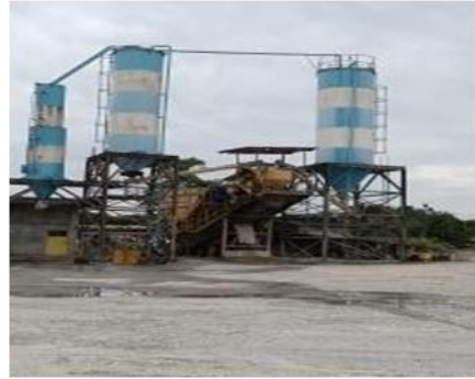
Gambar 1.3. Mesin Batching Plant
