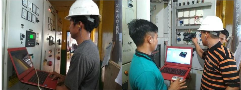
Gambar 2.18 Praktikum Input Data Program Deep sea electronics DSE 8610
