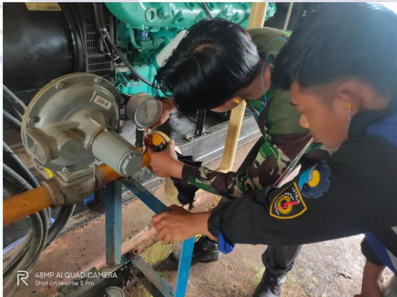
Gambar 2.17 Pembersihan *Regulator Gas Engine*
