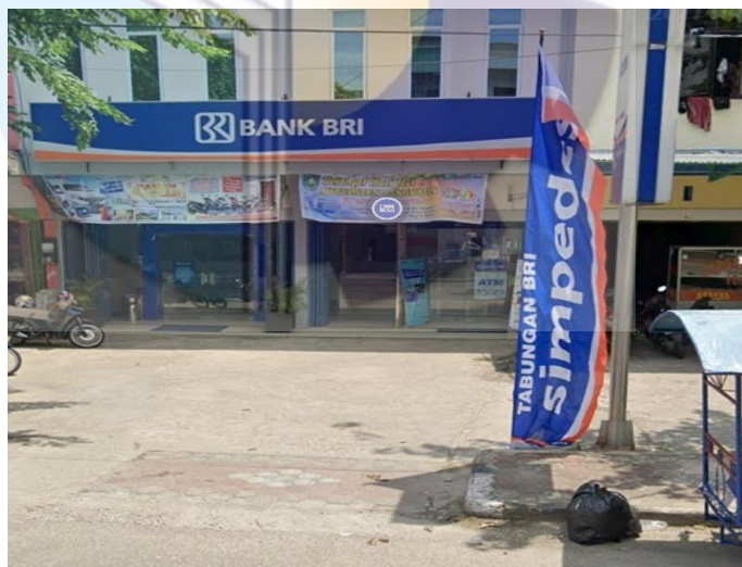
Figure 3.1 BRI sub branch office Bengkalis
