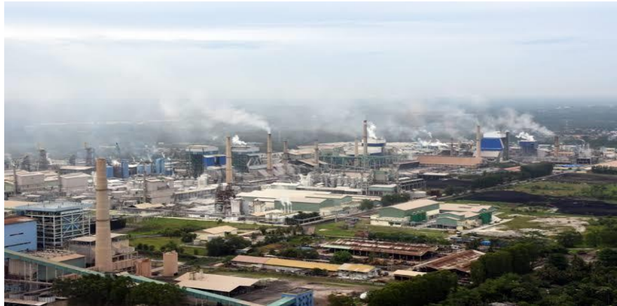
Figure 2.1 PT Indah Kiat Pulp & Paper Tbk Source: PT Indah Kiat Pulp & Paper Tbk - Perawang Mill
