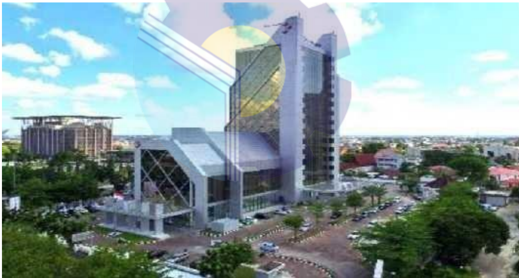
Figure 2.1 Dang Merdu Tower of Bank Riau Kepri
