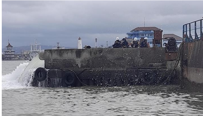
Gambar 2.33 Proses Pengeringan Kolam Graving Dock
