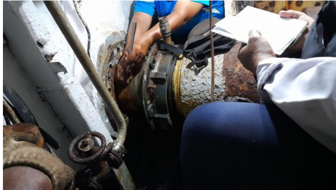
Gambar 2.15 Pengecekan Clearance Intermediate Shaft KMP Kirana III
