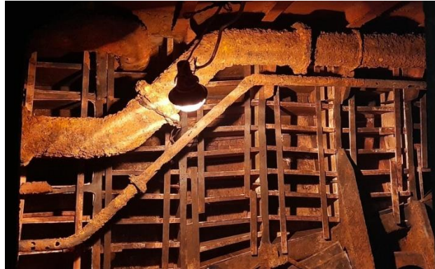
Gambar 2.23 Pengecoran Ballast Mati di KM Mulawarman
