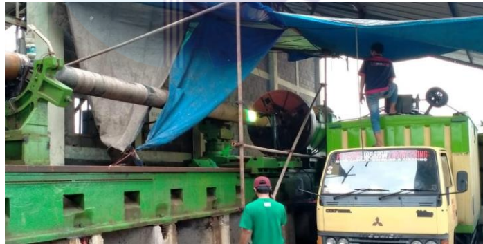
Gambar 2.19 Proses Spray Metal Shaft Propeller Kanan KM Kirana III
