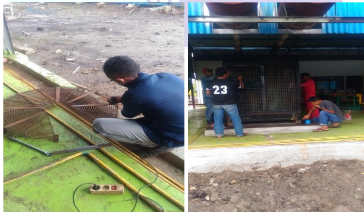
Gambar 2.2 perawatan radiator ( cooling ).
