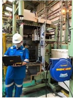
Gambar 2.10 Proses setting PLC diarea Pulp Dryer 3
