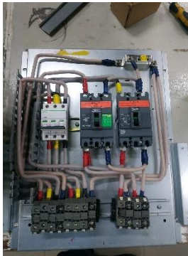
Gambar 2.19 Rangkaian Power Distributed Panel
