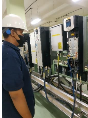
Gambar 2.20 Pengecekan VSD ACS-880
