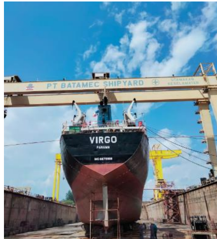
Gambar 1. 25 Graving Dry Dock
