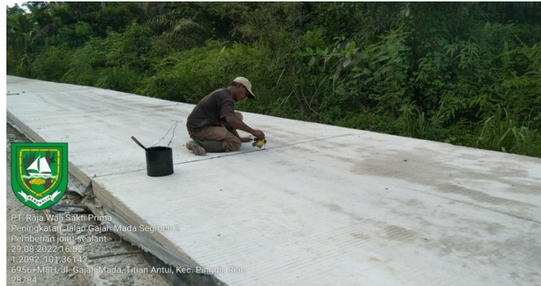
Gambar 3. 37 Joint sealant
