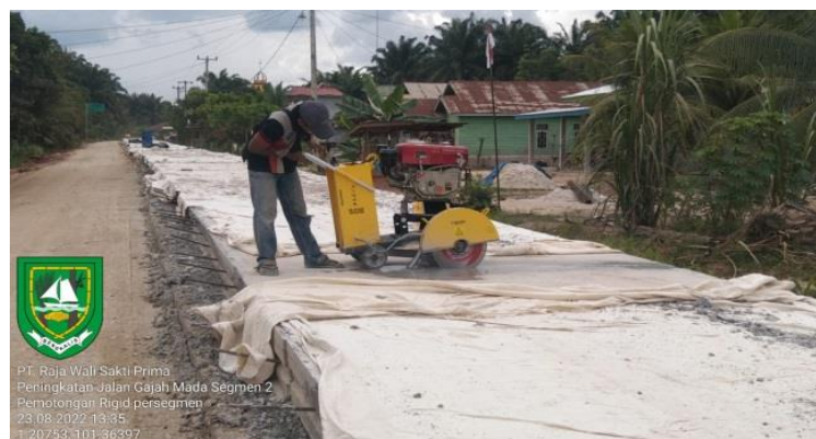
Gambar 3. 36 Cutting Beton
