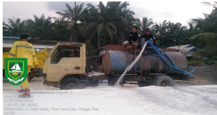
Gambar 3. 35 Curing Beton
