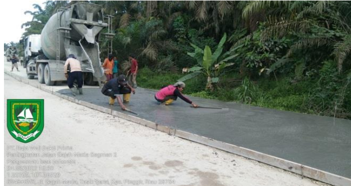
Gambar 3. 24 Pengecoran Lean concrete
