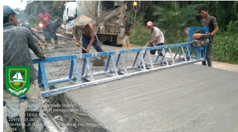
Gambar 3. 32 Truss Screed dan Beton Vibrator
