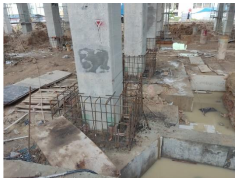
Gambar 3. 22 Pembesian Cover Column
