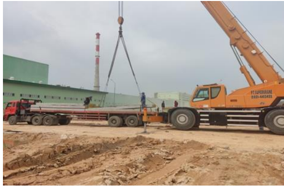
Gambar 3. 3 Unloading Spun Pile
