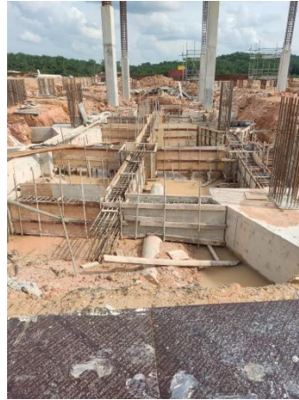
Gambar 3. 18 Pemasangan Bekisting Ground Slab
