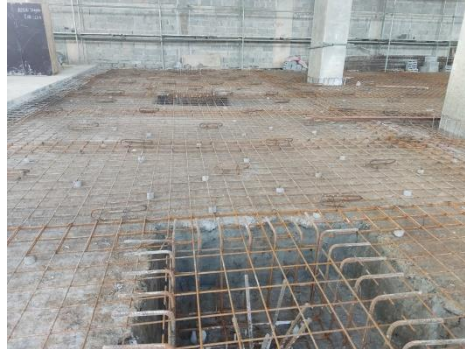
Gambar 3. 31 Pembesian Ground Slab
