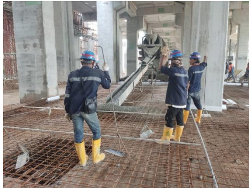
Gambar 3. 33 Pengecoran Ground Slab
