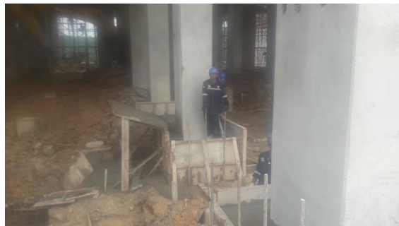
Gambar 3. 24 Pengecoran Cover Colomn
