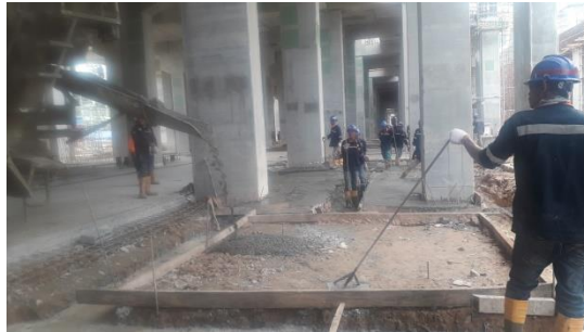
Gambar 3. 30 Pengecoran Learn concrete
