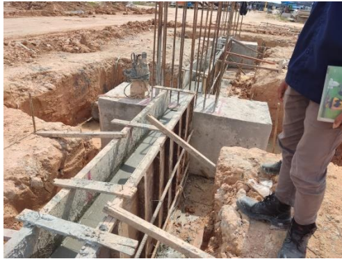
Gambar 3. 19 Pengecoran Ground Slab
