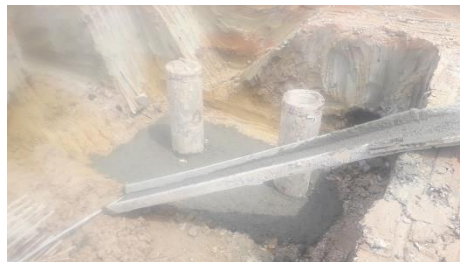
Gambar 3. 8 Pengecoran Learn Concrete
