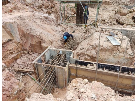
Gambar 3. 17 Pembesian Ground Beam
