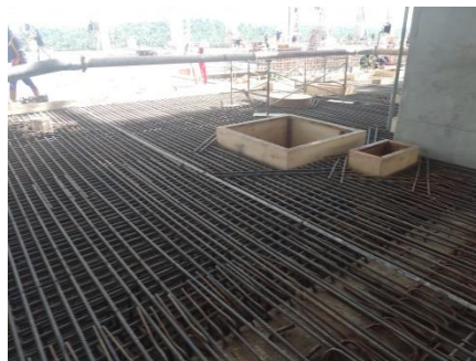
Gambar 3. 36 Pembesian Topping Slab
