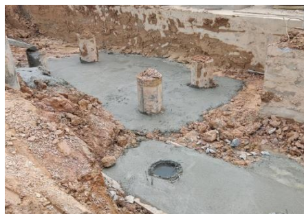
Gambar 3. 16 Pengecoran Learn Concrete
