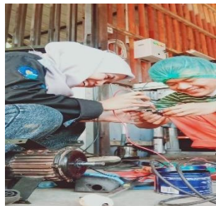
Gambar 2. 11: motor 3 phasa Sumber : Dokumentasi pribadi di PT.Cassia Co-op.
