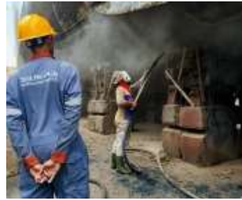
Gambar 3.2 Proses Sandblast
