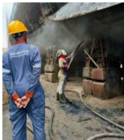
Gambar 2.14 Proses Sandblast
