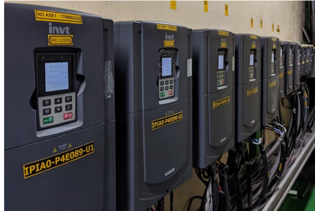
Gambar 3.3 Variable Speed Drive (VSD) GD 35 Series (Sumber: Dokumentasi di PT. Indah Kiat Pulp & Paper)
