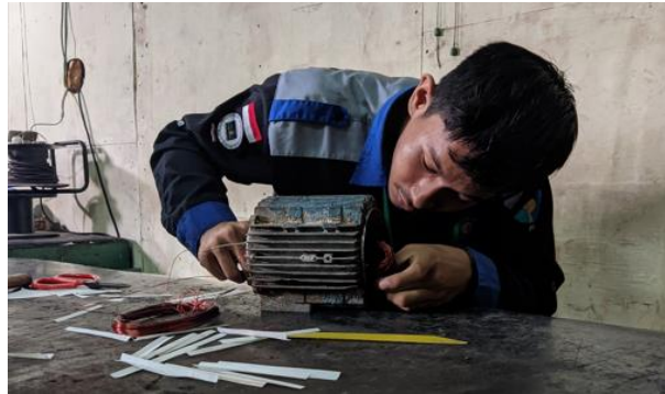
Gambar 2.18 Training Rewinding Motor 3 Fasa (Pemasangan Coil) (Sumber: Dokumentasi di PT. Indah Kiat Pulp & Paper)
