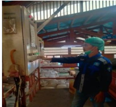
Gambar 2.6: Pengecekan Panel Casing (Sumber :Dokumentasi 2022)
