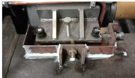
Gambar 2.43 Pemberian compound box chockfast
