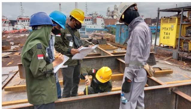
Gambar 2.6 Inspect T. Bulkhead Vert. Web. W20"x4"x9mm
