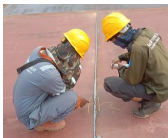
Gambar 2.15 Inspect welding join plat bottom
