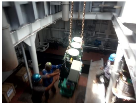
Gambar 3.10 Lifting OWS
