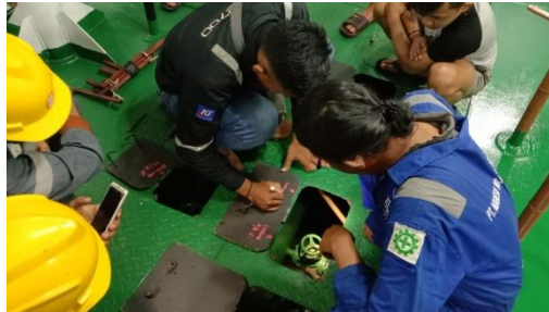
Gambar 2.20 Commissioning Piping System
