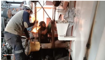
Gambar 2.38 Setting intermediate shaft
