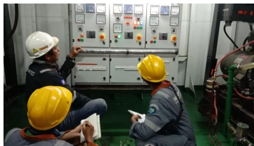
Gambar 2.26 MSB kapal Tugboat Hull No.1401
