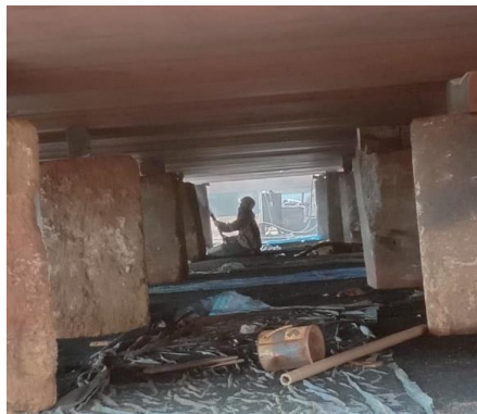
Gambar 2.11 Proses sand blasting
