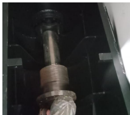
Gambar 3.14 Pemasangan kopleng as
