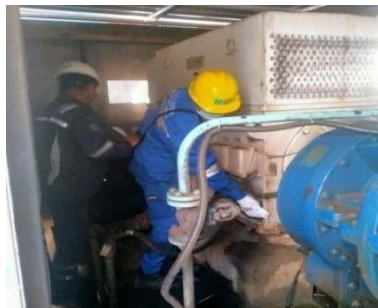
Gambar 2.37. PM Diarea Boiler Motor HPFF Unit 1
