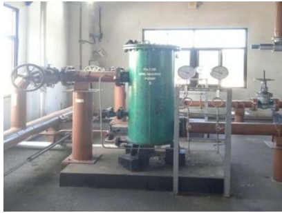
Gambar 2.31. Filter Unloading Pump 2 PLTU Tenayan (Sumber: Dokumentasi di PT PJB UBJOM PLTU Tenayan)
