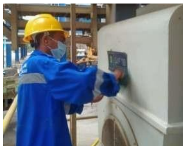
Gambar 2.34. PM Diarea Boiler Motor SAF 1B
