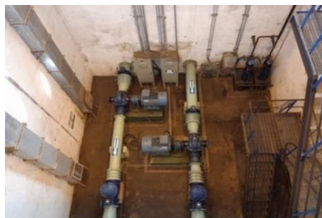
Gambar 2.16. Motor Water Intek Pump
