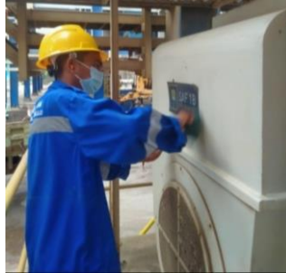
Gambar 2.34. PM Diarea Boiler Motor SAF 1B
