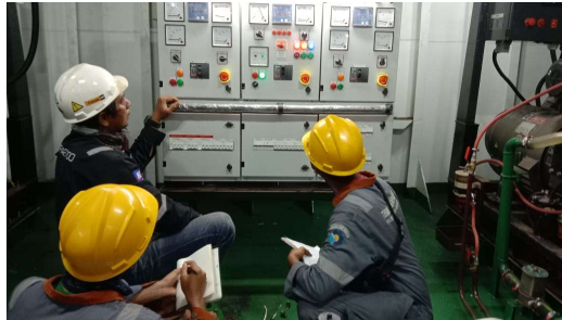
Gambar 2.25 MSB Kapal Tugboat Hull 1401
