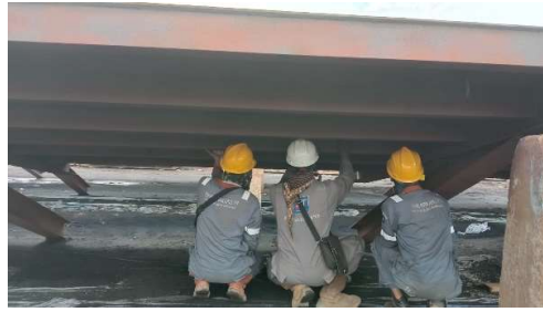
Gambar 2.60 Inspection Blasting
