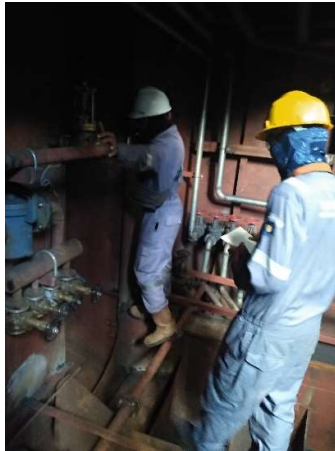
Gambar 2. 17 Pipe inspection
