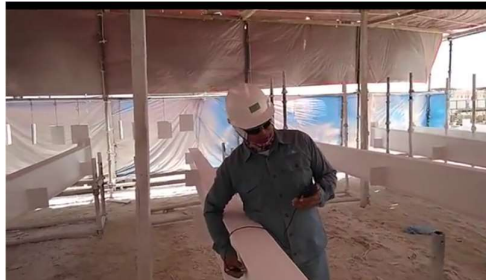
Gambar 2.57 Visual Inspection painting
