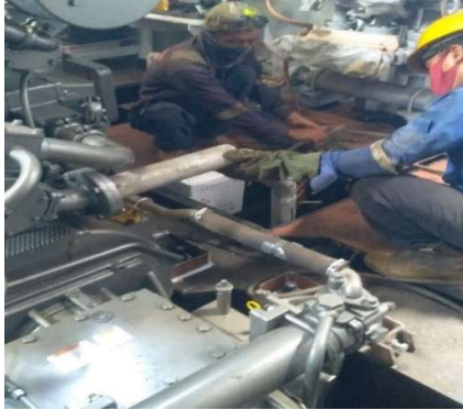
Gambar 2.39 Pemasangan pipa cooling system
