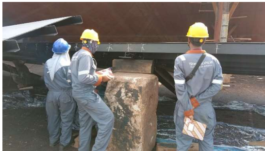
Gambar 2.5 Inspection welding side board
