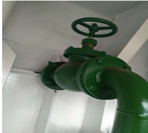
Gambar 3.13 Membuka Valve Overboard
