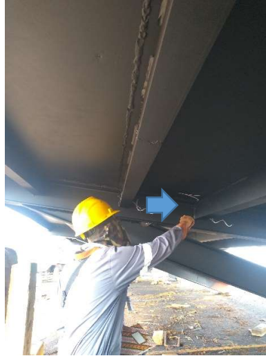
Gambar 2.16 Inspection welding bagian Sideboard
