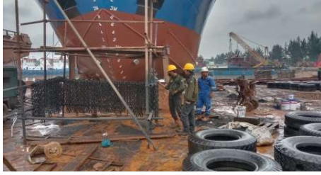
Gambar 2.62 Pengecekan akhir painting sebelum kapal launching
