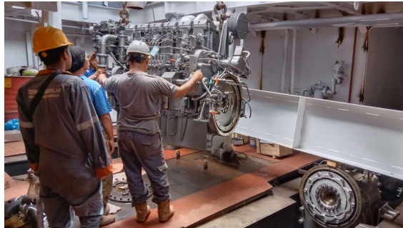
Gambar 2.30 Pemasangan Main Engine
