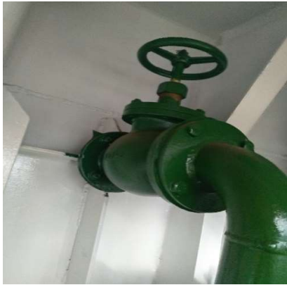
Gambar 3.8 Pipa Overboard dan SDNRV
