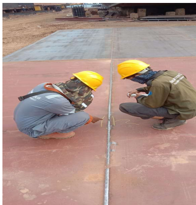
Gambar 2.13 Inspection welding Bottom Plat
