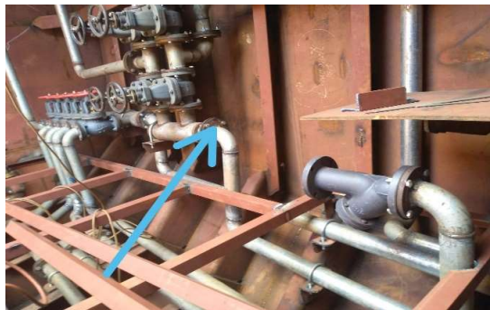
Gambar 3.3 Pipa Ballast
