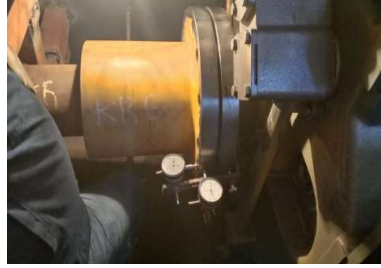
Gambar 2.28 Alignment Flange Shaft Propeller terhadap Gear box
