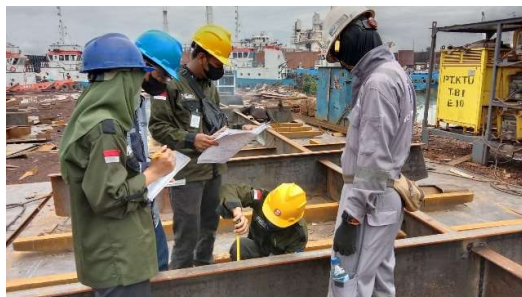
Gambar 2.6 Inspection Transversal Bulkhead
