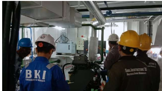
Gambar 2.54 Proses Load Test hull 1440
