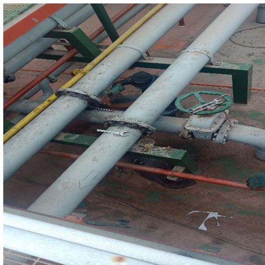
Gambar 2.27 ; Proses pergantian flange/sambungan pipa
