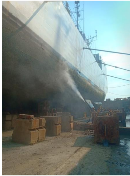
Gambar 2.2 Proses sand blasting lambung
