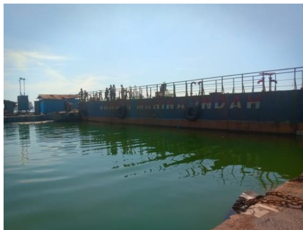
Gambar 3.8 Pintu Graving Dock
