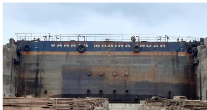
Gambar 3.2. Pintu graving dock
