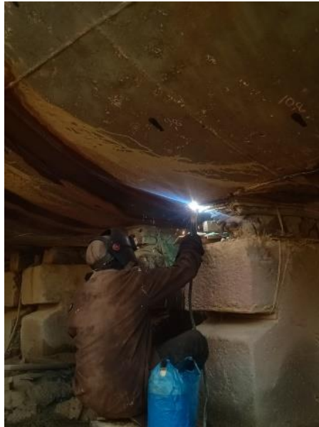
Gambar 2.13 Replating lambung bocor
