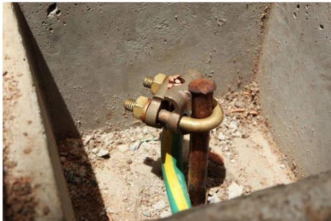
Gambar 3.1 Pemasangan Grounding
