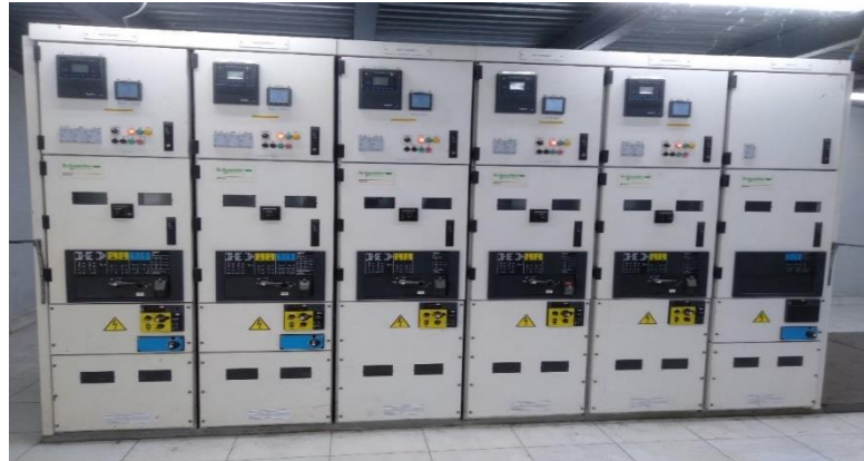
Gambar 3. 1 Panel MVMDP (Sumber: PT. WINA OLEO CHEMICAL, 2022)
