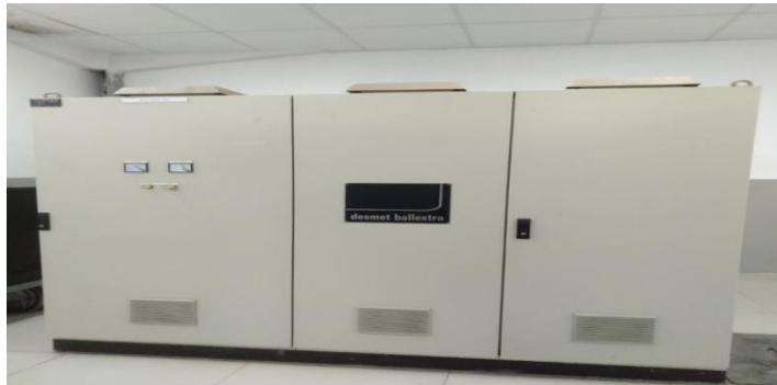
Gambar 3. 5 Panel PLC (Sumber: PT. WINA OLEO CHEMICAL, 2022)
