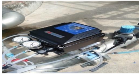
Gambar 2. 17 Positioner Kontrol Valve (Sumber: PT. WINA OLEO CHEMICAL, 2022)
