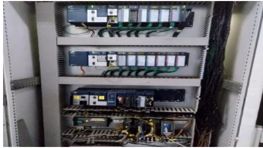
Gambar 2. 22 Panel Plc (Sumber: PT. WINA OLEO CHEMICAL, 2022)
