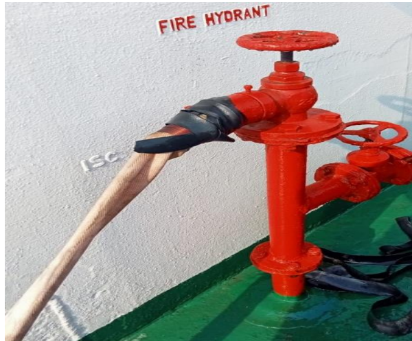
Gambar 2.24 Fire Hydrant
