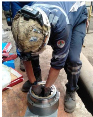
Gambar 4. 36 Pemasangan bearing kedalam housing
