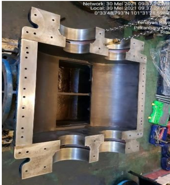
Gambar 4. 39 Install lower pedestal
