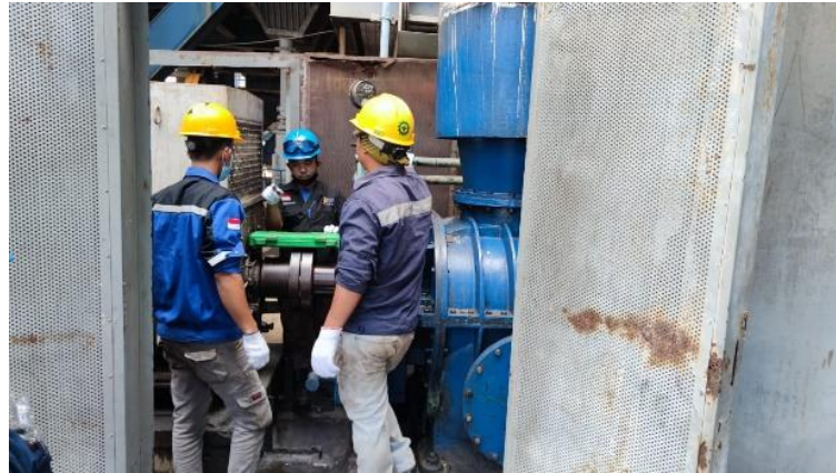
Gambar 2. 5 Corrective Maintenance pada High Preasure Feed Fan
