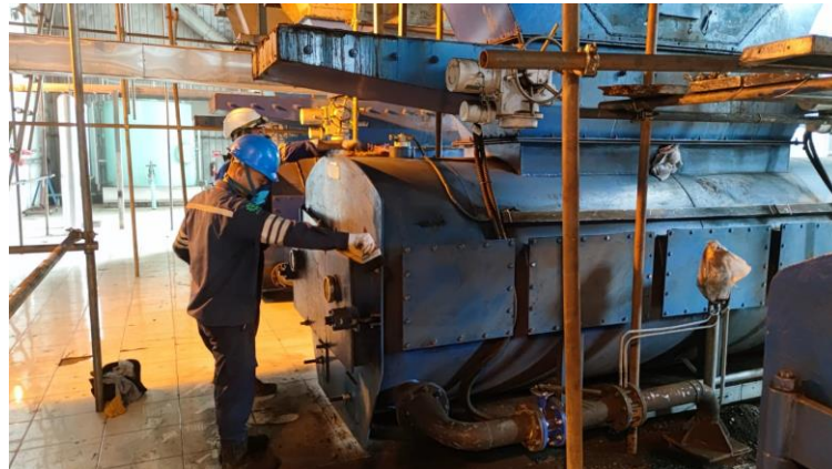
Gambar 3. 1 PM di area coal feeder
