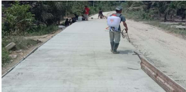
Gambar 3.41 curing beton
