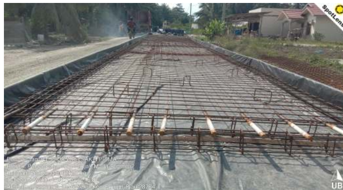
Gambar 3.33 Pemasangan crack inducer
