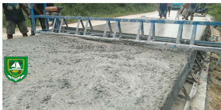
Gambar 3.39 Beton vibrator
