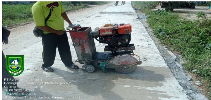
Gambar 3.43 cutting beton rigid
