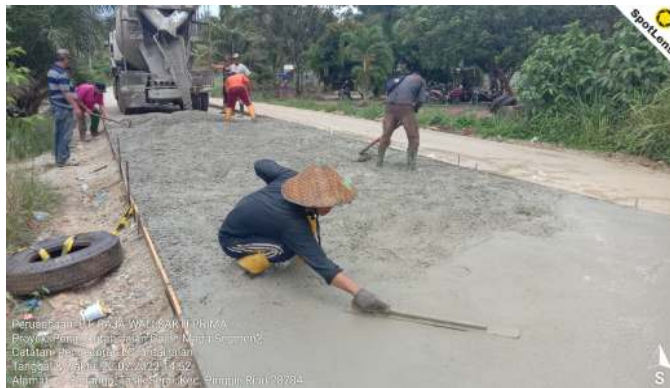
Gambar 3.27 Pengecoran lean concrete
