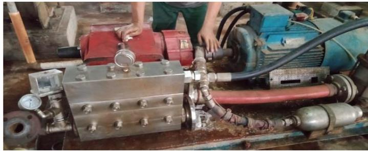
Gambar 4.1 Boiler *Feed Water Pump*
