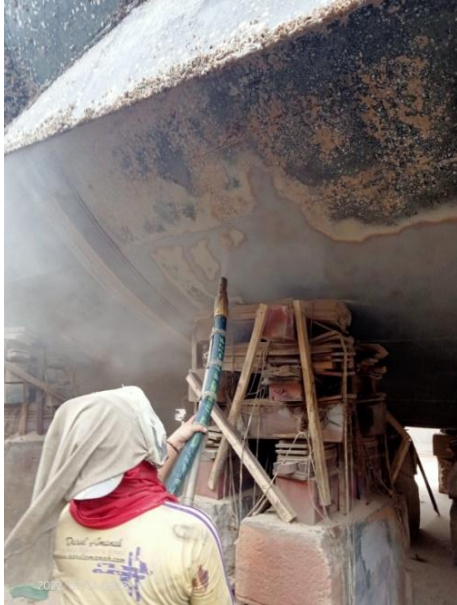
Gambar 2.11 proses rblasting
