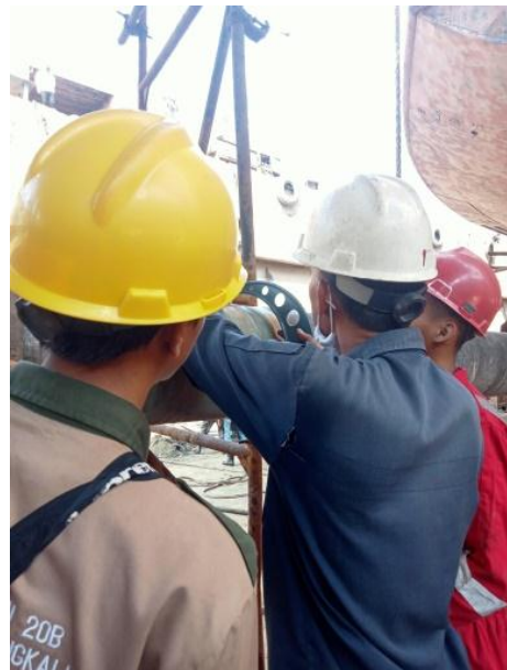
Gambar 2.24 pengukuran shaft propeller
