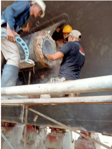
Gambar 2.23 pengukuran bantalan shaft
