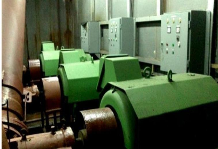
Gambar 1.9 Motor Pompa Graving Dock
