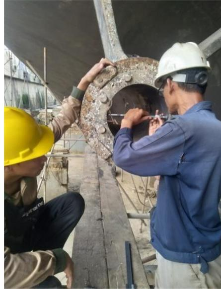
Gambar 2.12 pengukuran diameter v bracket
