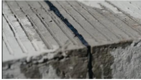
Gambar 4. 9 Pekerjaan Joint Silent
