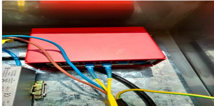
Gambar 4.5 OTB(Optic Terminal Box)
